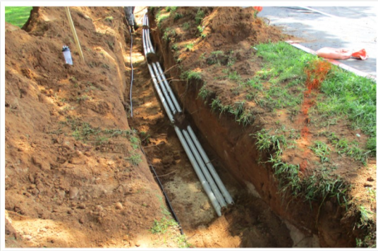
Installation of the electrical lines that had to be re-routed around the field.
