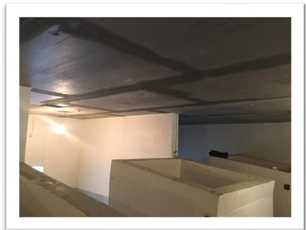
The above photo shows the install of the new stucco that has been applied to the ceiling.
